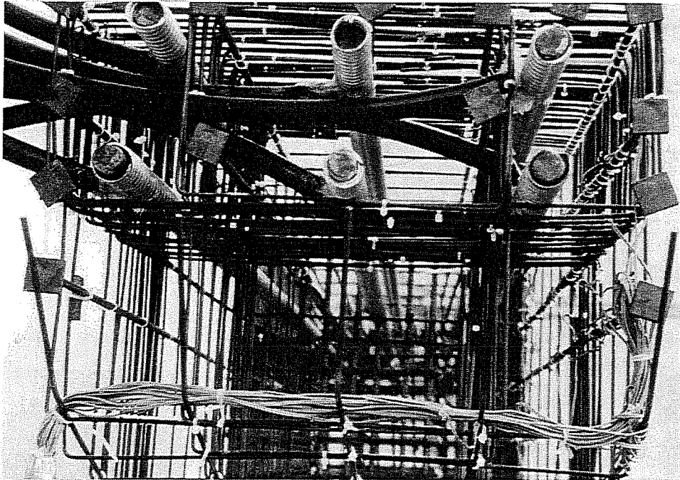
Figure 2.23 T-Headed Reinforcement in Model CO-PU-74S-TH-V
